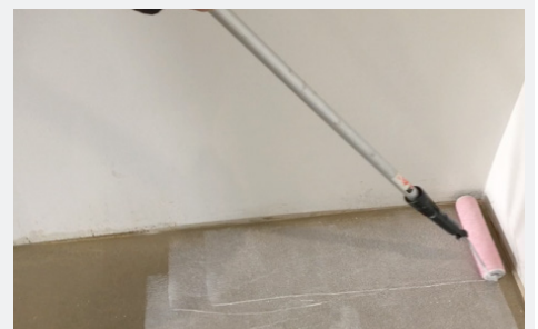
Fig 03: iTe SLURRY over VAPORiTe+PLUS
