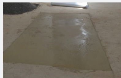
Fig 07: Finished bulked up coat
