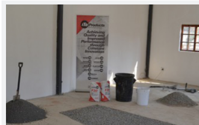
Fig 05: Levelled stone spread
