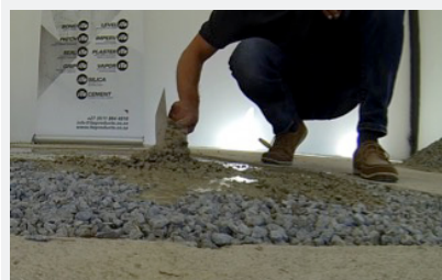
Fig 06: Trolling in LEVELiTe. Bulked up coat.
