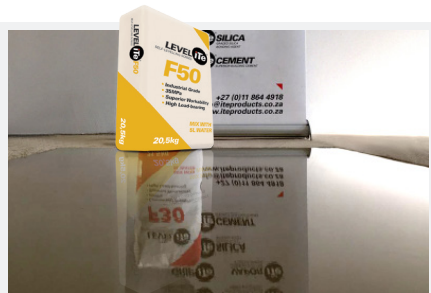
Fig 08: Final LEVELiTe coat
