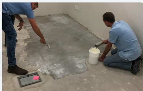
Fig 01: VAPORiTe+PLUS first coat
