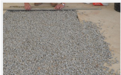
Fig 04: Stone spread in area to be filled
