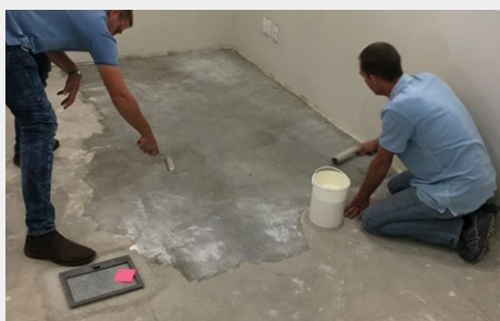
Fig 01: VAPORiTe+PLUS first coat
