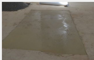
Fig 07: Finished bulkup coat
