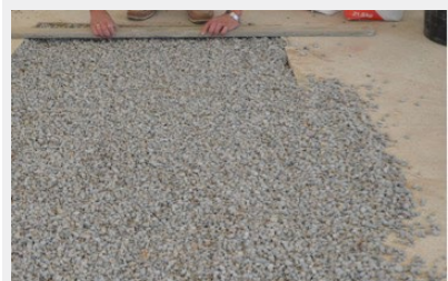
Fig 04: Stone spread in area to be filled
