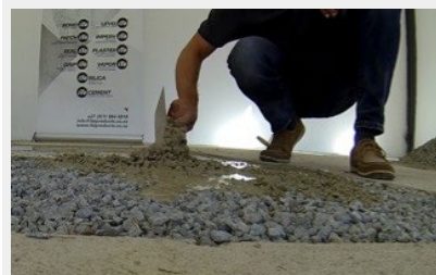
Fig 06: Trolling in LEVELiTe. Bulkup coat.
